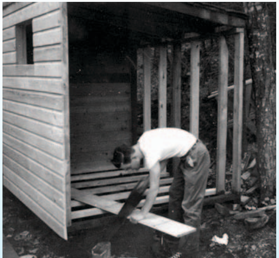
James Garvin building the tool shed
